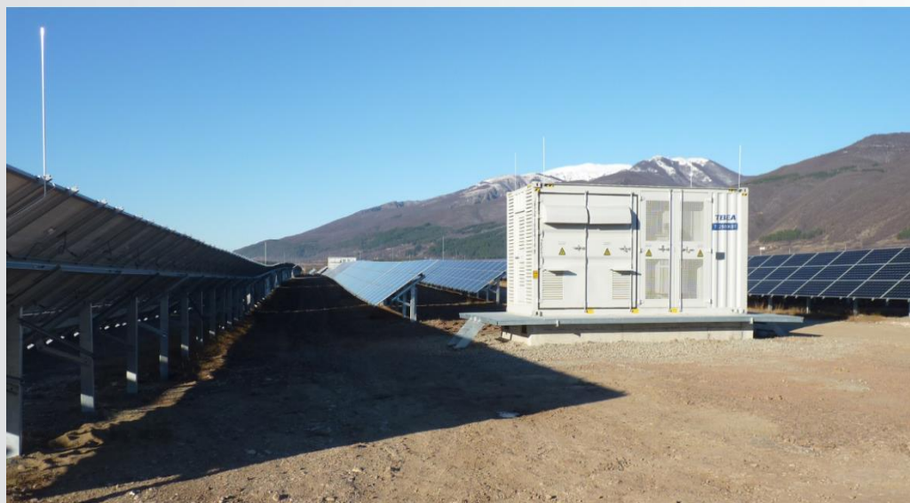
Bulgaria 25MW-Central Inverter+ MV Station Solution
